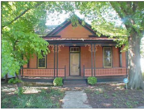
Painstakingly restored sawn-work is one of many unique features of this 2 bedroom*, 1 bath house that is thought to have been built much earlier than the 1915 date shown in the tax records. *The 2nd bedroom does not have a closet.
