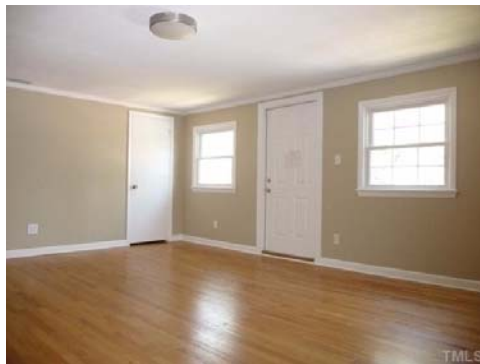
One of three upstairs bedrooms, the biggest has a non-functional exterior door that once led to exterior stairs that were later removed.
