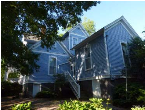
The old detached kitchen is now the office/studio/guest bedroom with a full bath. This is the view from the off street parking area accessed in the side yard accessible from N Bloodworth St.
