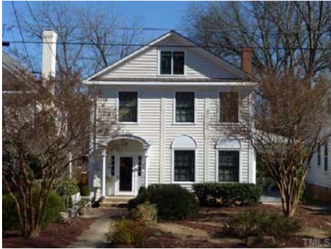
Unique character. Neo-Classical style with full-height pilasters, pedimented gable, arched hood, demi-lunes over 6/6 windows. So states the nomination of the Mordecai Place neighborhood as a national (not local) historic district.
