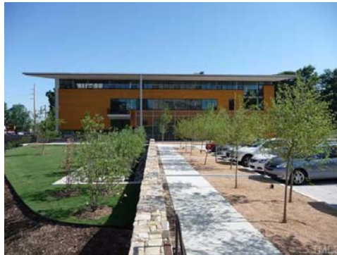
As part of the nearby Blount Street Commons, the new HQ for the state architects' association (NC AIA) offers a gathering place for neighborhood meetings including those addressing the City of Raleigh study of the Blount-Person Street corridor.
