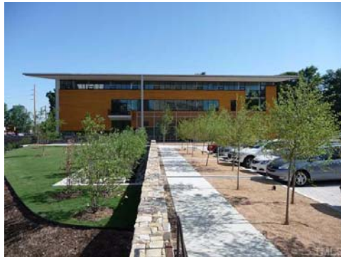
As part of the nearby Blount Street Commons, the new HQ for the state architects' association (NC AIA) offers a gathering place for neighborhood meetings including those addressing the City of Raleigh study of the Blount-Person Street corridor.
