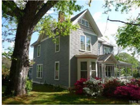
Designated as a Capital Tree, this magnificent Oak shades the Queen Anne style home that has a carved sunburst in the porch gable, and alternating bands of scalloped and rectangular slate roofing shingles.
