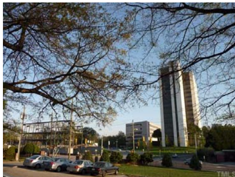
Walk to work at the nearby state government offices shown here across the street from Peace College and towering over the steel skeleton of the new AIA HQ. Catch a bus to NC State or the R-LINE circulator service in and around the downtown.
