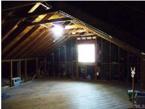
The upstairs walk-in attic provides lots of storage.
