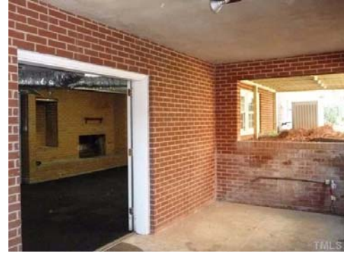
A covered patio under the Sun Porch opens through double-doors into the lower level Den. This and the partially finished connecting spaces could be reconfigured as in-law suite or efficiency apt with the addition of a lower level bath and/or kitchen.
