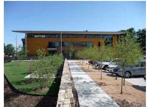
Across from the Peace University, the new NC AIA Center for Architecture and Design is a venue for community meetings and celebrations. It is part of the Blount Street Commons development providing live-work-play options that include Gallery C.
