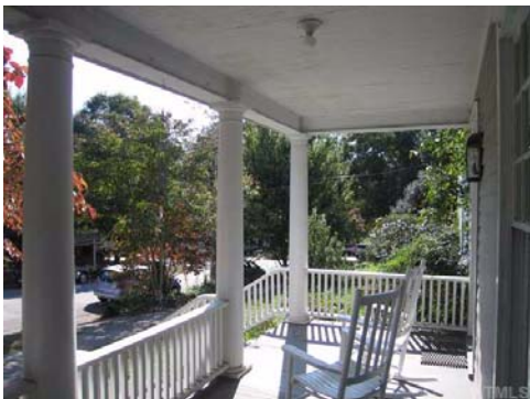
The front porch is nicely elevated.
