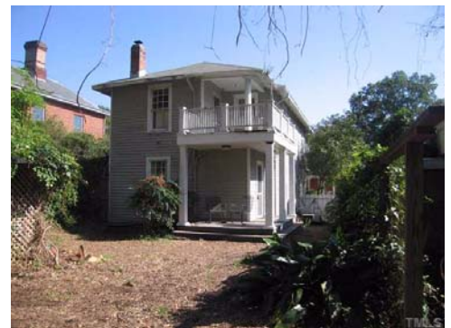
The compact 0.08 acre lot offer lots of opportunities for lawn, garden and patio. Recently removed, climbing ivy had covered much of the house and yard.
