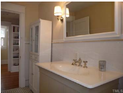
Nicely accenting the old house character is the new gracefully shaped, enameled cast iron vanity counter top.
