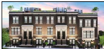
* Hargett Place Rowhomes (19 under construction)
