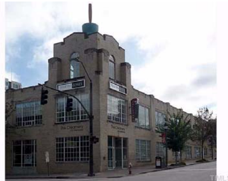
The Glenwood South entertainment district, three blocks to the south, includes an adaptably reused dairy building and lots new including condos and a hotel. State government offices and museums border the district to the east.
